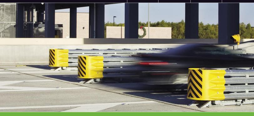
The TRACC™ Family of crash cushions includes TRACC™, a narrow Test Level 3 cushion; SHORTRACC™, a narrow Test Level 2 cushion; FASTRACC™, a narrow Test Level 3 crash cushion with additional capacity for head-on impacts up to 70 mph (113 kph). The WIDETRACC™ is available in varying lengths, widths, and test levels (per design speed). It can be config-ured for any appropriate wide application.
